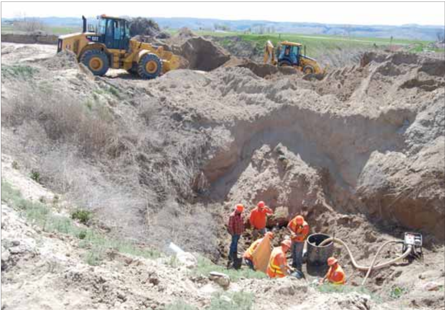
Construction crews have been working on installing new culverts and irrigation piping under U.S. Highway 95 between Homedale and Marsing before irrigation water was turned on Monday. Workers are also digging deep to install drainage culverts before the resurfacing of almost nine miles of the highway. U.S. 95, closed since April 5, should reopen Thursday.
